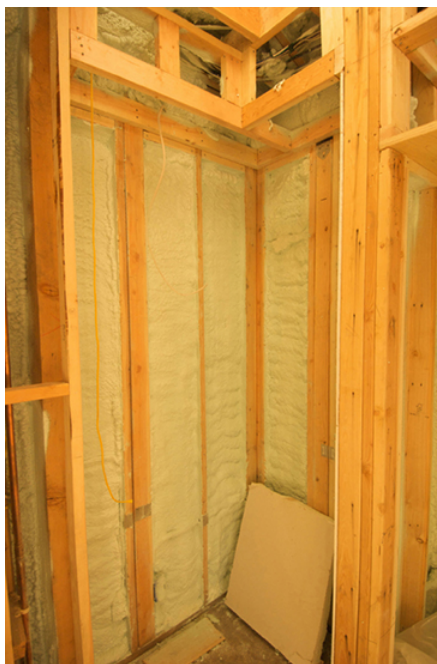
Figure 1.7.2: Insulation is used to limit the conduction of heat from the inside to the outside (in winter) and from the outside to the inside (in summer). (credit: Giles Douglas)
