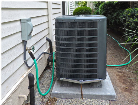
Figure 4.6.4. A photograph of a heat pump (large box) located outside a house. This heat pump is located in a warm climate area, like the southern United States, since it would be far too inefficient located in the northern half of the United States. (credit: modification of work by Peter Stevens).
