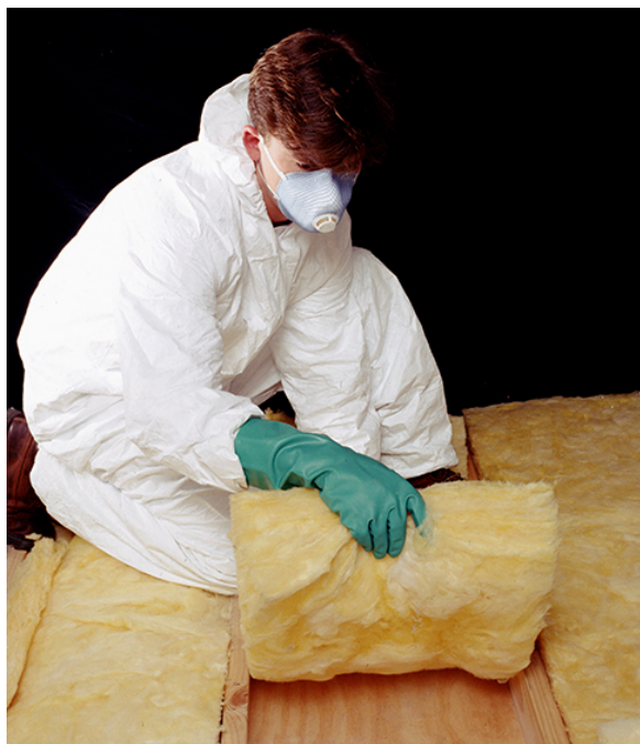
Figure 1.7.5: The fiberglass batt is used for insulation of walls and ceilings to prevent heat transfer between the inside of the building and the outside environment. (credit: Tracey Nicholls)
