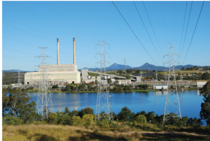
Figure 7.7.5: (a) Schematic of an electrostatic precipitator. Air is passed through grids of opposite charge. The first grid charges airborne particles, while the second attracts and collects them. (b) The dramatic effect of electrostatic precipitators is seen by the absence of smoke from this power plant. (credit b: modification of work by “Cmdalgleish”/Wikimedia Commons)
