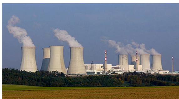
Figure 4.3.2: The heat exhausted from a nuclear power plant goes to the cooling towers, where it is released into the atmosphere.
